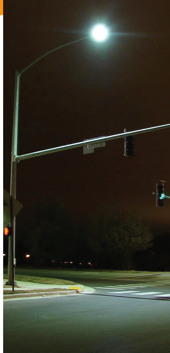
A study prepared by PG&E and Energy Solutions in Oakland, CA reported the comparison between a 121-Watt HPS and 78-Watt LED luminaires. As shown above, the LED's CRI (up to 80) is much higher than the HPS(30) and allows for more crisp visibility.
